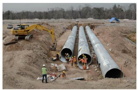
The materials for 2.1 metres multi-plate culvert were delivered to the site and assembly is currently underway
