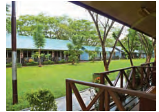
Clean employee housing at the Kelanis River Facility.
