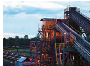
The Kelanis River Facility recently added an additional crusher to expand capacity to around 55Mt.
