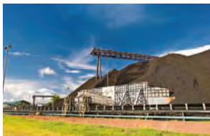
11. Coal stockpiling at Kelanis
