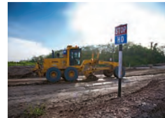
Grading the hauling roads for safety and efficiency.
